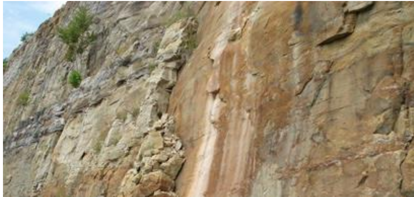
Fig.3: Plane failure
