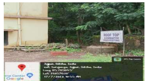
Roof Top Rain Water Harvesting
